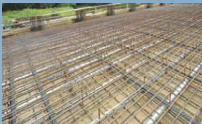
Reinforcing steel and post-tensioning ducts in a haunched slab bridge.
