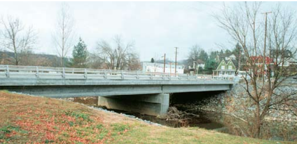
The use of HPC in the Richlands Bridge allowed the number of beams per span to be reduced from seven to five. All photos VDOT unless specified otherwise.
