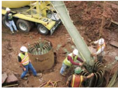
Self-consolidating concrete was used in the drilled shafts of the Route 28 Bridge over Broad Run.
