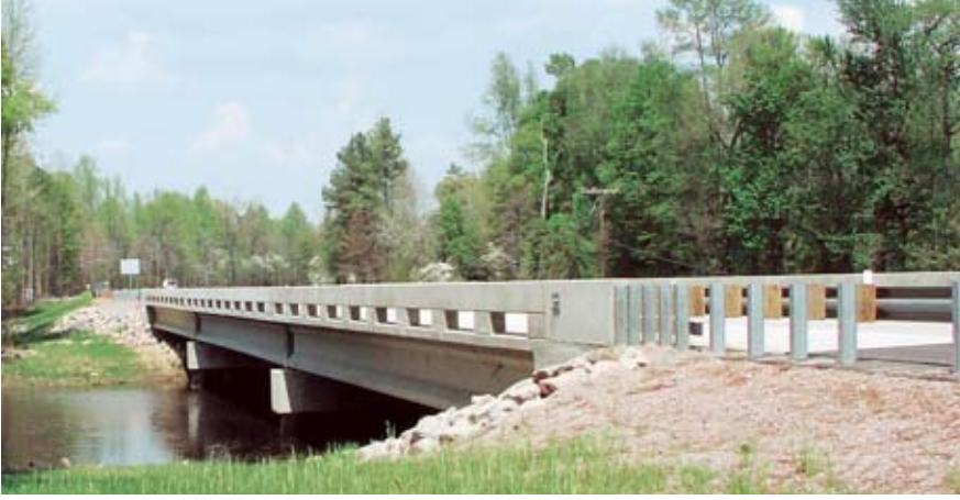
The Route 106 Bridge over the Chickahominy River was the first use of lightweight high performance concrete.
