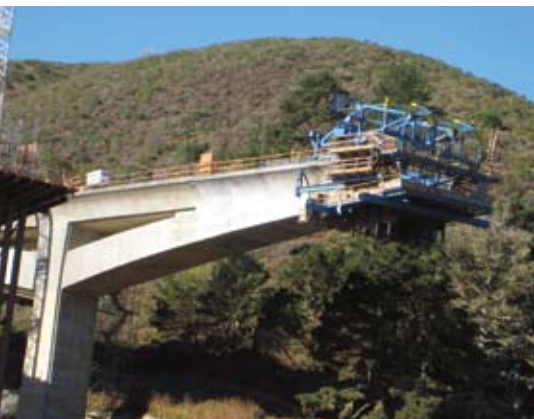
Form travelers are used to construct the main span cast-in-place segments over the environmentally sensitive valley below.
