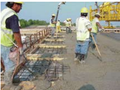
A 4-in.-thick topping was cast on the beams before onsite erection.
