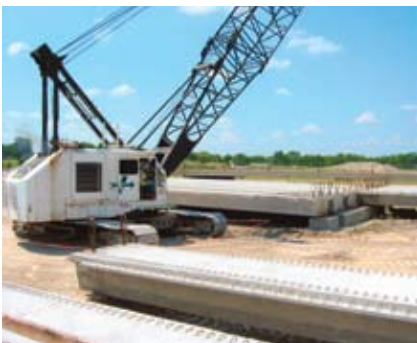
Beams were preassembled for casting the deck.
