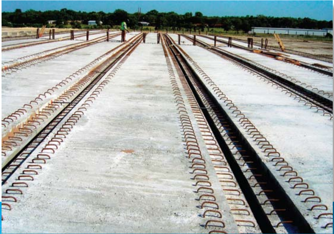
Beams were preassembled for casting the deck.
