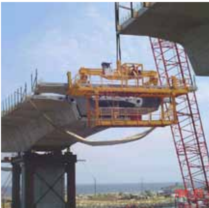
Segment erection was performed using the balanced cantilever construction method.
