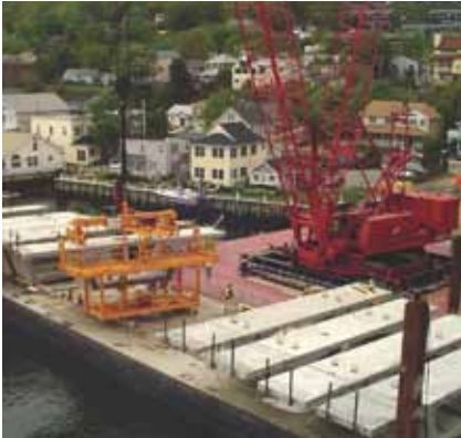
Segments were shipped from the precasting plant to the bridge site by barge, and were erected using a ringer crane and specially designed spreader beam. The stressing and installation platform was attached to the segments prior to lifting.
