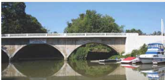
The newly widened bridge provides better functionality and the same historic appearance as the original. Although local groups were wary, feedback has indicated that the results have been well received, and the project has been perceived as a success. All photos: ENTRAN PLC.
