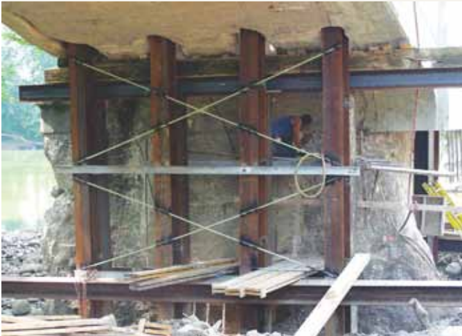
A temporary support system was placed under the arch on either side of the pier during the construction process.
