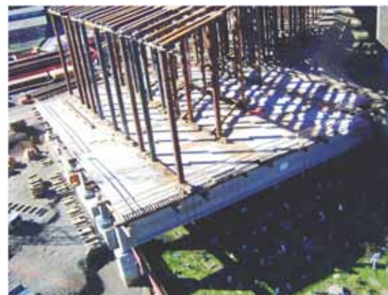
Placing concrete in the soffit of the box girder.
